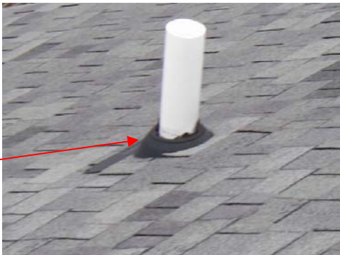
Sample – roof repairs: Torn shingle (wood exposed) Deteriorated vent boot
