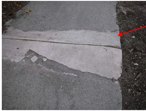
Sample – raised side walk, attempted repair (broken edge)
